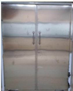
Lead Lined (X Ray Room) Door
